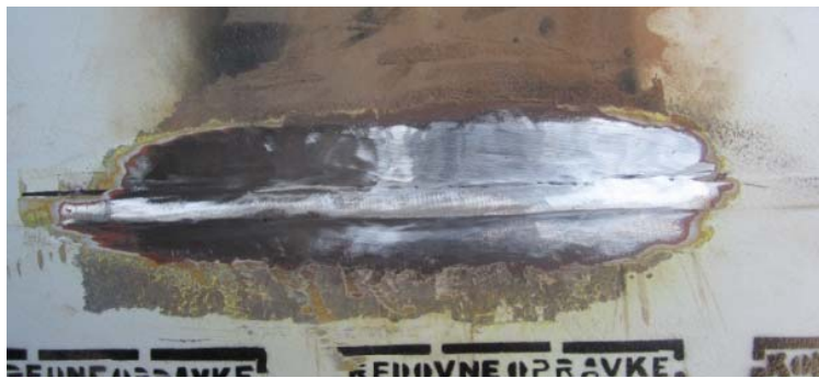
Picture 6. – The repair of welded joint
