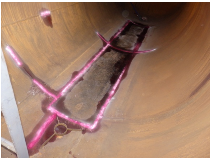
Picture 10. – Additional sheet metal repair zone
