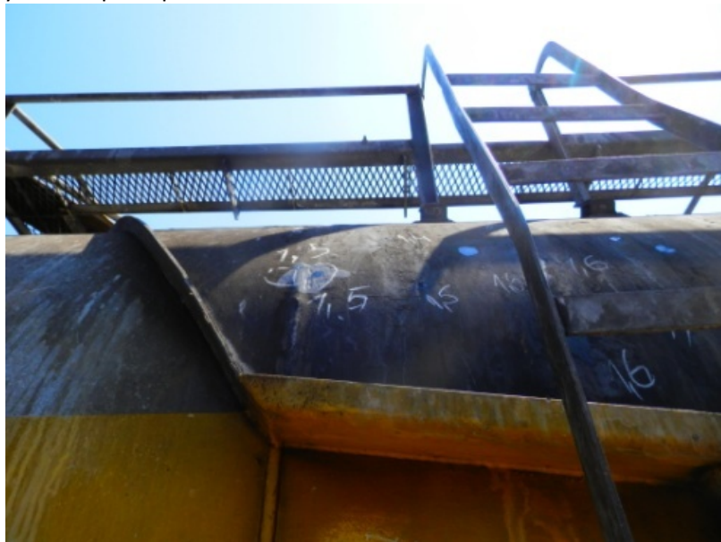
Picture 1. – Some of the wall thickness measurement points
