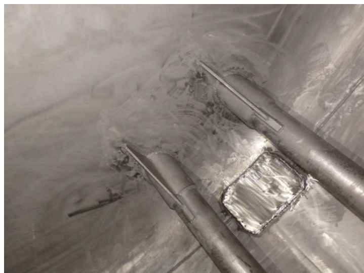
Picture 4. – The patch in the place of the crack
