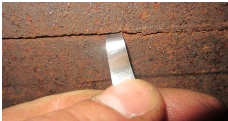
Picture 5. – Part of the incomplete weld
