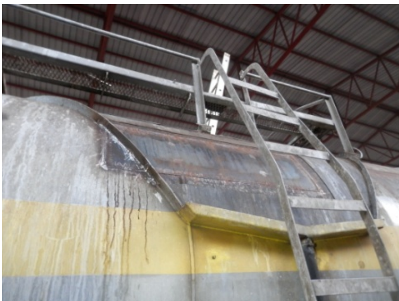
Picture 2. – Replaced segment around the dome
